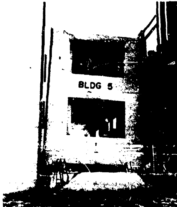
Figure 4.55 Post-Elder, (Item 26) Station 3.1.1, close-up of Building 5, first floor collapsed. Pressure level: Elder, 20 psi.
